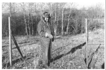
Fence posts are made from three 5 1/2-ft. long 2 by 4's nailed together to form a triangular-shaped base
