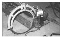
Mackey's antique circular saw cut through logs up to 28 in. in dia. and could also make horizontal cuts.
