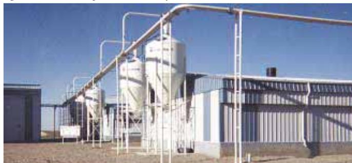
To make the blower pipes they bought 20-ft. lengths of drill stem pipe, sandblasted them and painted them white, then clamped them together.
