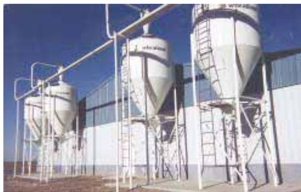
Pipes lead from each bin back to the distributor which is located near the farm's feed mill.
