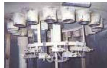
We used steel tubing to support the blower pipes about 20 ft. off the ground and mounted them in cement footings.
