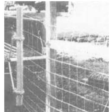
An A-shaped puller is chained to a pickup, tractor or come-along to stretch the fence.
