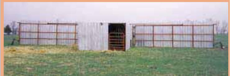
Shelter consists of a 24-ft. long enclosed barn and two 24-ft. long, 8-ft. high wings that fold out to form a windbreak. Note gate at end of barn.
