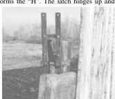
down on a bolt. To hold the gate you simply flip it down on either side of the gate.
