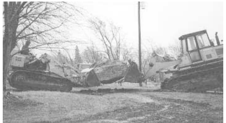
A pair of crawler tractors with buckets were used to load the rock onto a semi trailer for transport.
