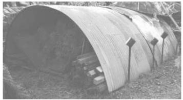
Low-cost shed was made by placing two bin halves side by side on ground and using steel posts to keep the sides from spreading out.
