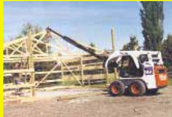
to 30 ft. Lift capacity depends on the size of the loader and the angle of the lift.
