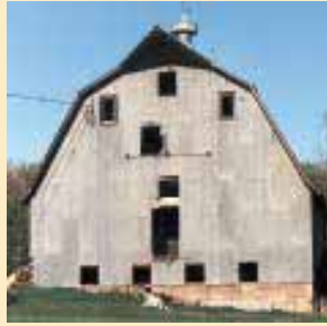
The McKinnon's turned this dilapidated gambrel-roofed barn into a beautiful modern home.
