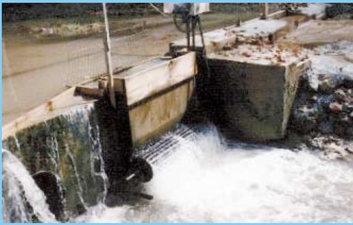
**Dam across creek is 4 ft. high, 20 ft. wide and 18 in. thick. Water falls 33 in. onto a 12-in. dia. turbine that drives a modified Delco car alternator.**
