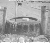
Center of tire is filled with concrete level with bottom bead on tire. After the concrete has hardened Bach installs the stand pipe, float system, and overflow.
