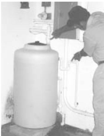
Marley set up a 65-gal. tank to mimic an aquarium. Once water has been "treated", it's pulled from there into the household pressure system.
