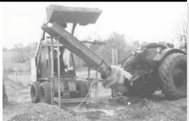
Lloyd Armstrong, Sunderland, Ontario: "Here's an idea I came up with when we needed to pour a lot of concrete in our barn and cow yard. I built a dump chute that feeds directly into our tractor-mounted 1/3-yard cement mixer. I put the correct amount of cement in with a pail and then use a skid steer to dump in one bucket full of 3/4-in.
