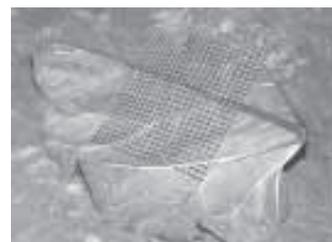
To start, lay out a rhubarb leaf with the veins up. Wire mesh is embedded in the concrete for added strength.
