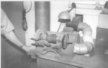
Richard Cox, Jacksonville, Ill.: "Grinding jobs are a lot cleaner ever since I installed a vacuum system to carry dust and small grindings out through my shop wall. I used a
