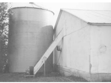
Engler put a 2,400-bu. bin at the end of his hog barn. To get hot air from the barn attic to the bin, he made a 16-in. sq. duct from plywood and connected it to the intake side of an aeration fan that he mounted inside the bin.
