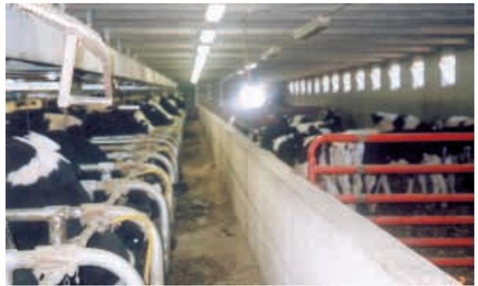
With clear span roof panels there are no interior support poles to get in the way. All equipment is hung from the ceiling, which makes cleaning easier.
