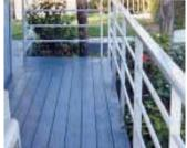
Tongue-and-groove 2 by 8 boards can be used as deck flooring.
