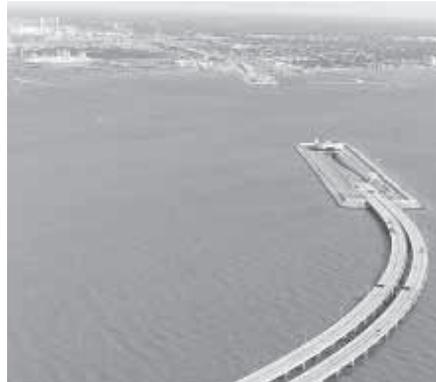
This bridge between Sweden and Denmark "disappears" under the sea so ships can still travel normally overhead.
