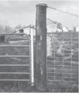
Post welded to gate is 2 in. below and 1 ft. above it, which puts the hinge bolts further apart. This stops gate from sagging.
