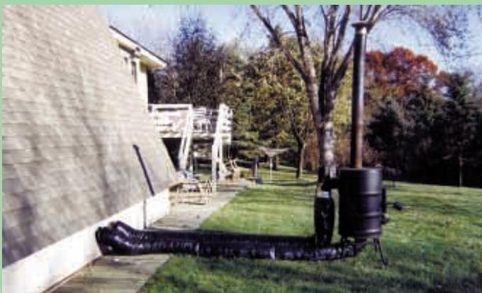
Tad Schreiner's wood burning stove sends heated air through insulated air ducts into his shop, which is located under the living space in his house.
