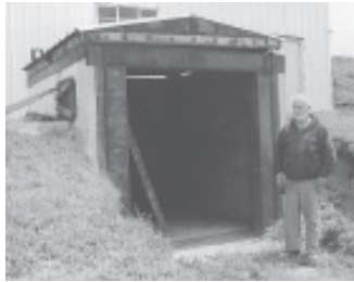
Clair Wilson dug this 8-ft. high firebox into the ground next to his shop. It has a hinged roof that can be raised to drop 7-ft. logs inside with a loader tractor.
