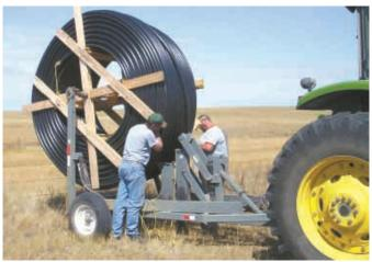
Tractor-mounted pasture plow cuts up to 2 ft. into ground to lay in pvc water pipe. The 1 1/2-in. pipe Hagen uses comes in 6,200-ft. rolls.
