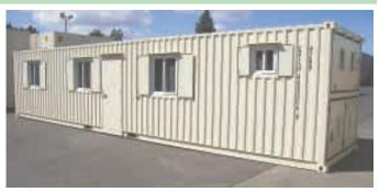
California firm turns steel shipping containers into temporary or even permanent housing. The 8-ft. wide buildings are up to 40 ft. long and can be connected together.
