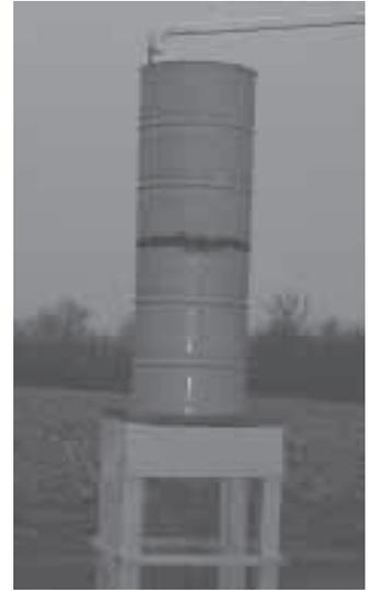
**Garden "water tower" eliminates the need for a pump. It was built by welding together two 55-gal. barrels.**
