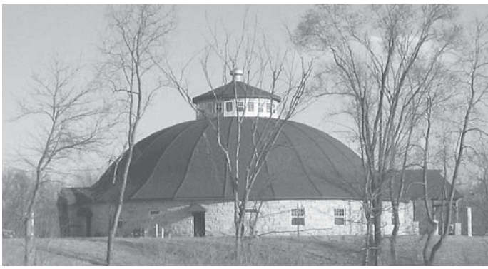
Dick Schwab built this 100-ft. dia., 8,000 sq. ft. round barn with the help of volunteers.
