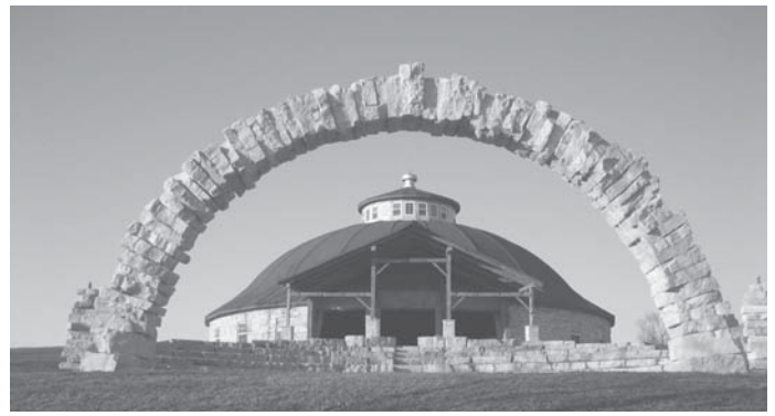
Built to host community events, there’s a 500-seat stone amphitheatre outside and a large, mortarless stone arch.
