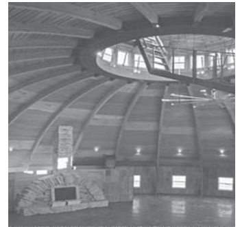
Interior ceiling is covered with 12,000 sq. ft. of home-sawn cherry and maple. Note massive 12-ft. tall stone fireplace.
