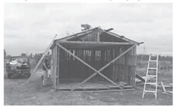
Frank Pye's 12 by 20 by 7-ft. shed has a floor made from 18 pallets. The shed walls are two pallets high.
