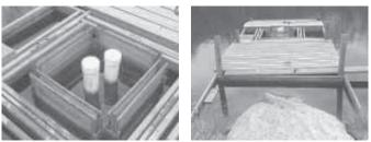
Kelsey Hydro System intake pipes and filter trap (left). Intake tank catches water coming off dam. Photos courtesy BrianWilcox
