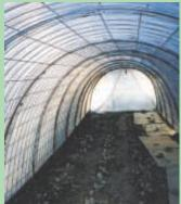
Lengths of 1-in, dia. plastic tubing are duct taped over every joint where the panels come together.
