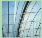
Panels are wired together at 2-ft. intervals where they meet. Wire ties are covered with duct tape to keep from tearing the
