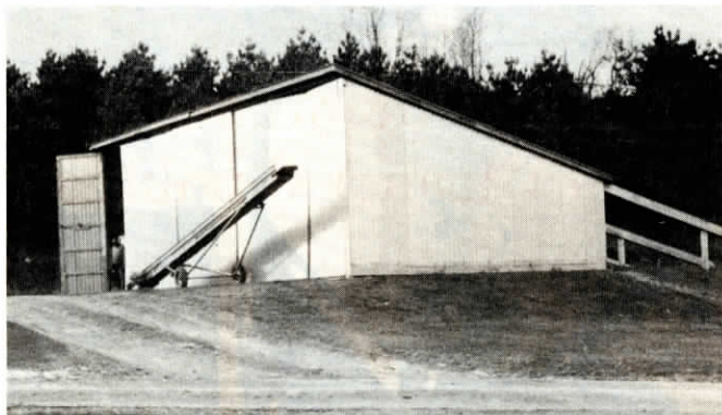
Rafters extending to ground serve as "track" for sliding roof sections.
