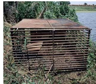
Beaver barriers made of steel bars, are used to enclose pvc overflow pipe.
