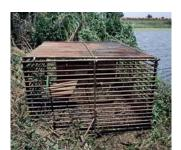
Beaver barriers made of steel bars, are used to enclose pvc overflow pipe.
