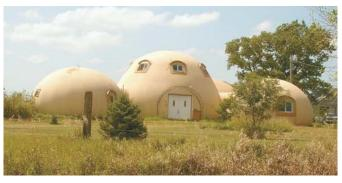
"Home domes" were created using airforms – big polyvinyl balloon-like shells inflated with air. Main dome is 32 ft. in dia. by 20 1/2 ft. tall.
