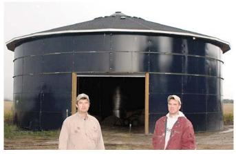
Todd Cole turned an old 62-ft. dia. Slurrystore into feed and machinery storage by putting a roof on it, and installing a 15-ft. wide by 16-ft. high door.
