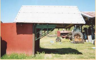
Rolling roof on well house allows James Padgett to pull up a bad well without having Entire back wall opens up for full access to well and pump.
