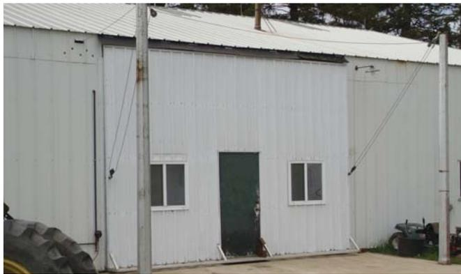
In the closed position, walk-through door and windows result in easier access and better lighting.
