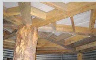
He used corrugated side-wall steel to create a curved roof over root cellar stairway (left). Post and beam roof structure supports second floor.
