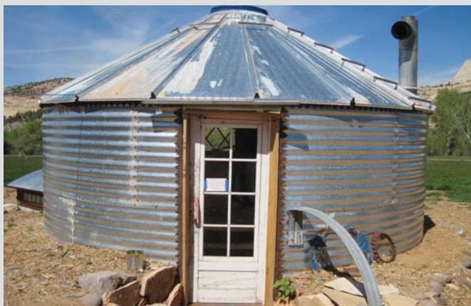
Scott Brodie built this 2-floor combination root cellar-storage shed out of an 18-ft. dia. corrugated steel bin, installing a white entrance door on front.
