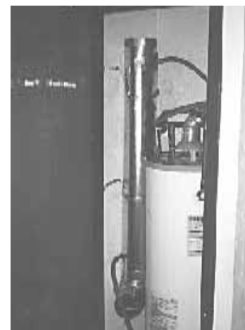
Cozy Heater mounts on side of any hot water heater and plumbs easily into the water lines.
