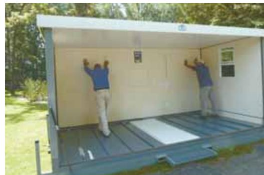
Once the shelters are in place, the 26-ga. steel-sided walls can be easily erected by 2 or 3 people in just a few minutes.
