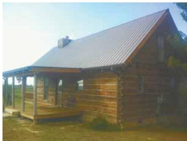
Concrete logs look like real hand-hewn logs but don't have the problems associated with wood such as warping, settling, twisting, and rotting.
