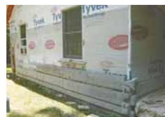
Concrete logs are 2 by 10 in. and 8 ft. long, with rebar inside to prevent the logs from cracking.
