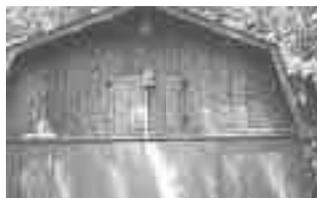
wide, 20-ft. long mini-barn. I used one section of the track and lag screwed it to a 2 by 4 board. A 4-ft. door rolls along the track. (Burney S. Jackson, 725 E. 116th St., Carmel, Ind. 46032 ph 317 846-3166)
