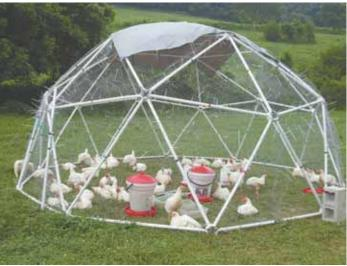
Thanks to the connecting hub design, one person can assemble the frame for a 16-ft. dia. Zip Tie Dome within a couple of hours.
