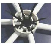
Dome's struts slip into holes on 4-in. dia. pvc hub. Zip ties slip through holes in struts for a secure connection.
