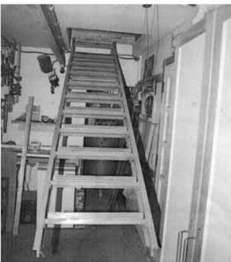
Upper end of ladder is hinged to one side of loft opening. Cables attached to side of ladder run up through ceiling and over pulleys to a bundle of old window weights. Weights are balanced so ladder floats up or down easily with one hand.
