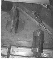
Upper end of ladder is hinged to one side of loft opening. Cables attached to side of ladder run up through ceiling and over pulleys to a bundle of old window weights. Weights are balanced so ladder floats up or down easily with one hand.
