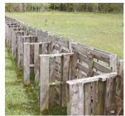
Pallets are used together at right angles.
