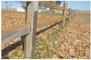
Loran Bauer uses steel posts to repair his split rail fence. He drives the post into the ground next to a weakened upright and then screws it in place.
