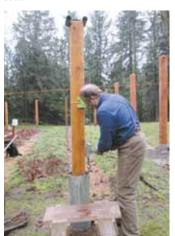
Come-along is used to pull metal duct out of hole, leaving landscape fabric in place.
