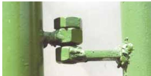
A simple nut-bolt combination can be used to make a sturdy gate hinge.
