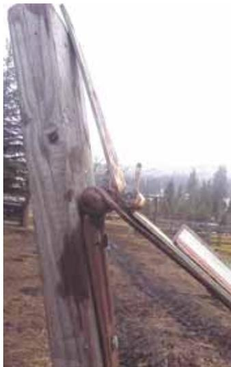
Hinges bolt together on 2 by 4 to provide leverage against wood posts.
