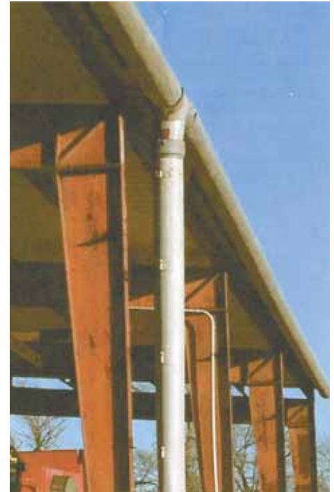
Leo Bottoms used 8-in. aluminum furrow irrigation pipe to make this rain gutter system for his 75 by 150-ft. shed. The gutter downspout empties into an underground pipe that runs to a nearby pond.
