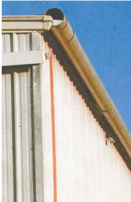
Leo Bottoms used 8-in. aluminum furrow irrigation pipe to make this rain gutter system for his 75 by 150-ft. shed. The gutter downspout empties into an underground pipe that runs to a nearby pond.
