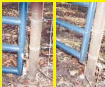
from sagging and makes it easy to keep it closed when there are no animals inside the pen. The bottom of the gate post simply slips over the top of the bracket. In addition, the same bracket can be welded to a "T" and driven into the ground to keep gates open and prevent sagging.
