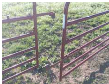
Tube gate latch system uses the weight of the gate to "cup" it and keep it straight.
